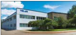
Williston, VT, U.S.A. Velan Valve Corp., Plant 3
