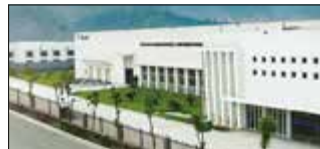
Suzhou, China Velan Valve (Suzhou) Co., Ltd.
