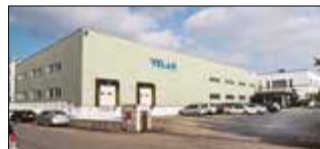
Ansan City, South Korea Velan Ltd., Plant 2
